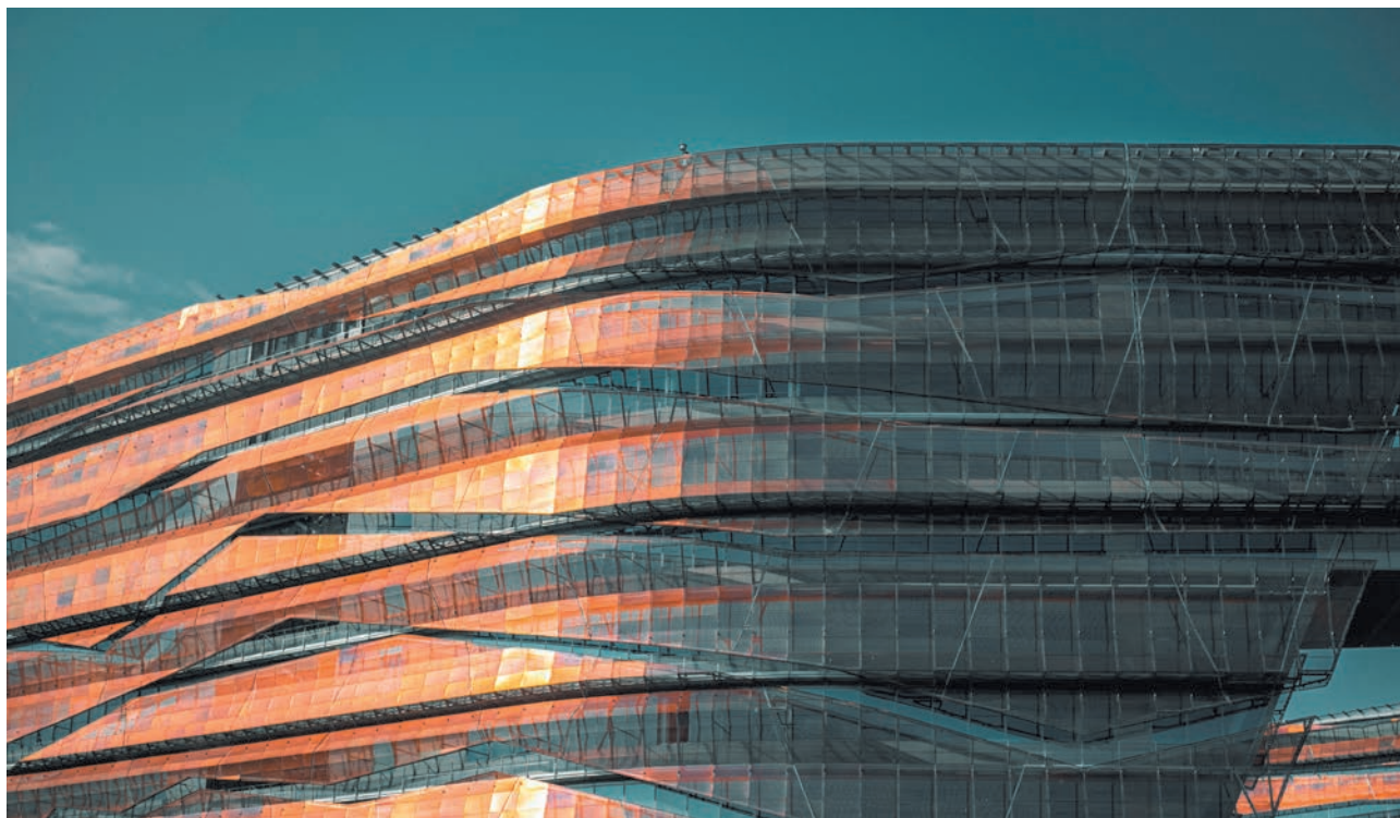
ENI Headquarter - Rooftop, terrasses et espaces extérieurs Milano, Italia Pedestal System - Pedestal Prime® e New Maxi NM
