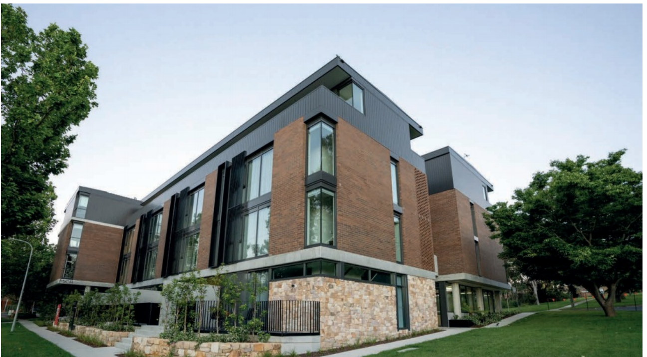
MICA (Middle of Campbell) – Rooftop, terrasses et espaces extérieurs Campbell, Australia Pedestal System – New Maxi NM
